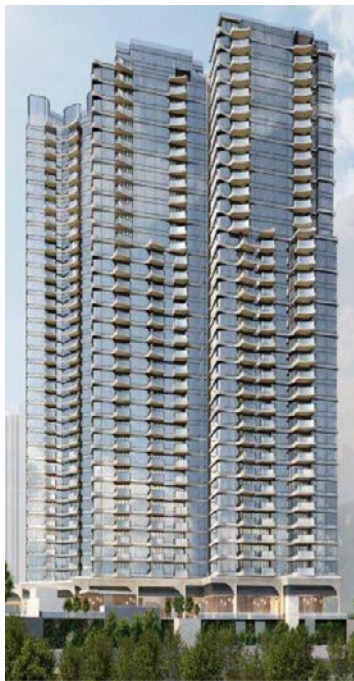
2. Deep Water Pavilla at MTR Wong Chuk Hang project (CSI – 15%) Presales ongoing
