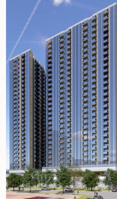
5. Lai Sun Yuen Long Center Redevelopment to commence in late 2026 (CSI – 50%)
