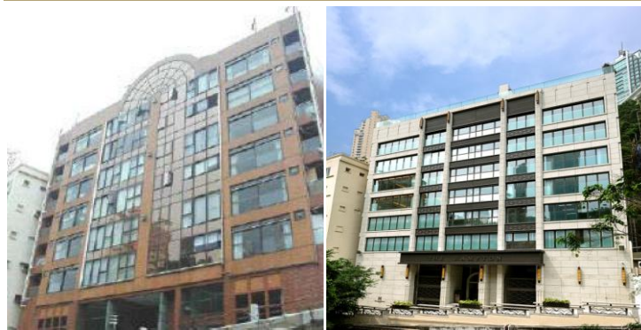
Exhibit 9: The Hampton before and after its makeover
