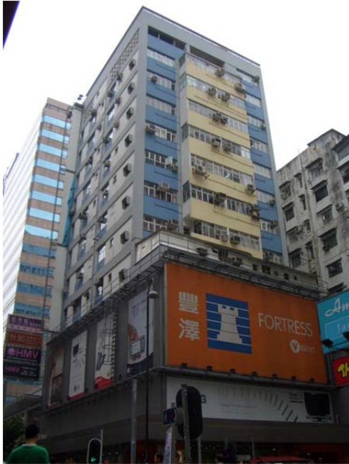
Exterior – before renovation
